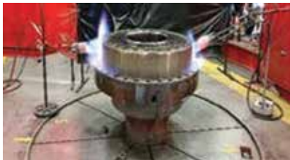
Heating with Gas Flame.
