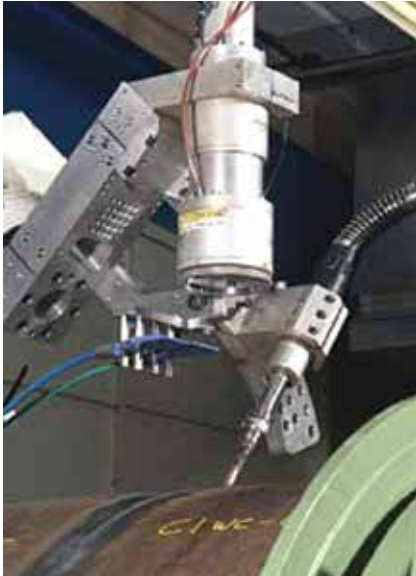
Fig.4a. Nd:YAG laser - MAG hybrid process being developed for land pipeline girth welding. Picture of the welding head
